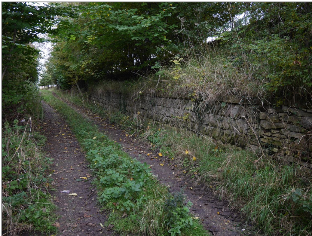
Figure 9b Looking north from the road along carriageway in stone revetted cutting
