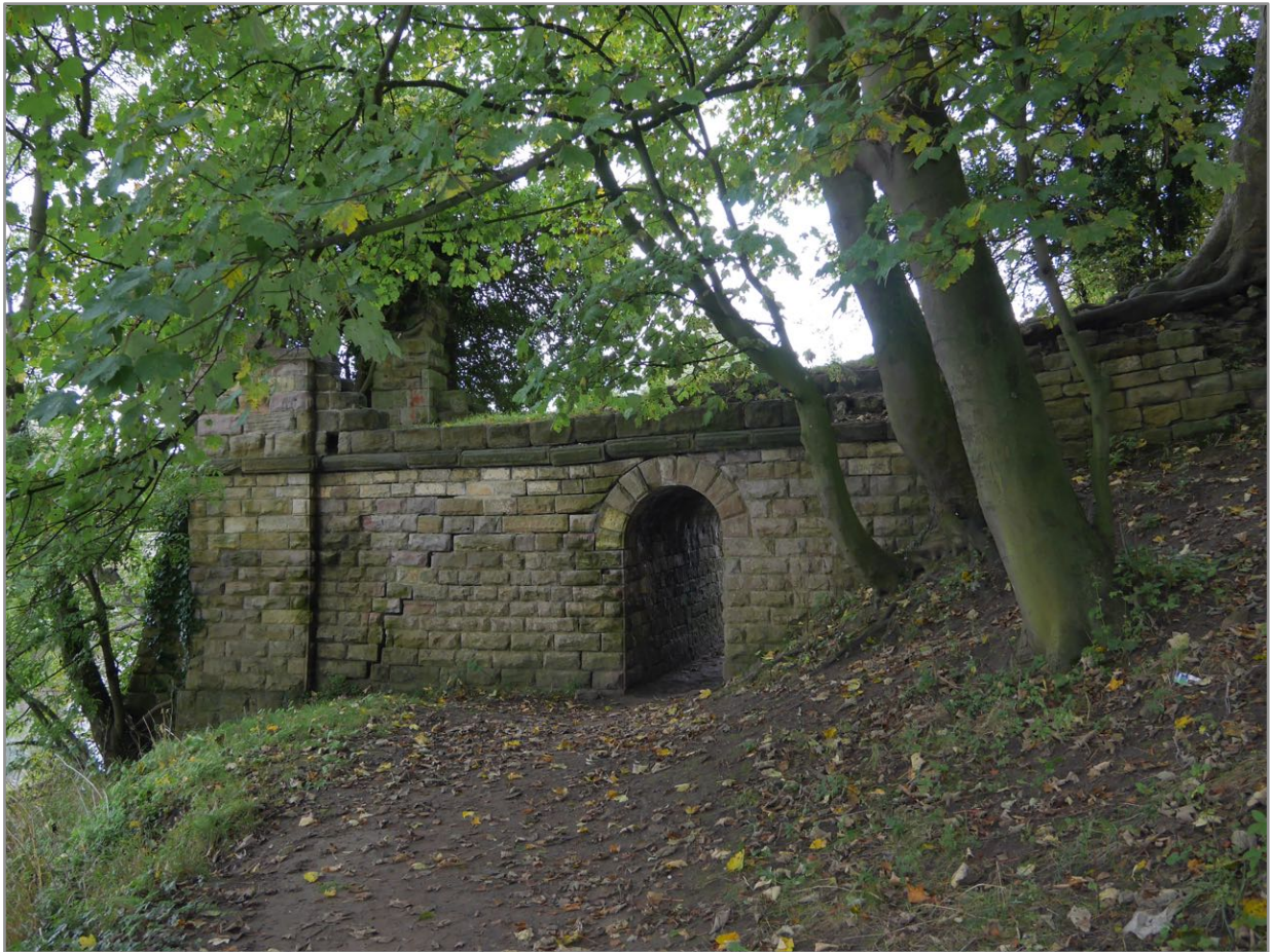
Figure 8 Remains of stone bridge abutment on south bank of River Wharfe
