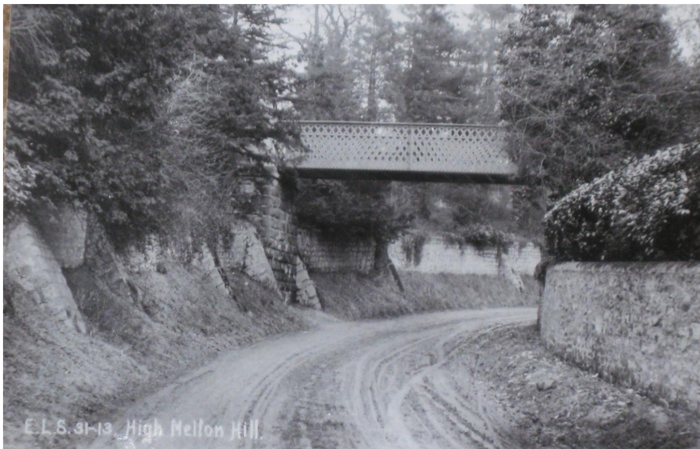
Figure 14 - Photograph of walkway from pleasure grounds to Melton Warren (undated)
