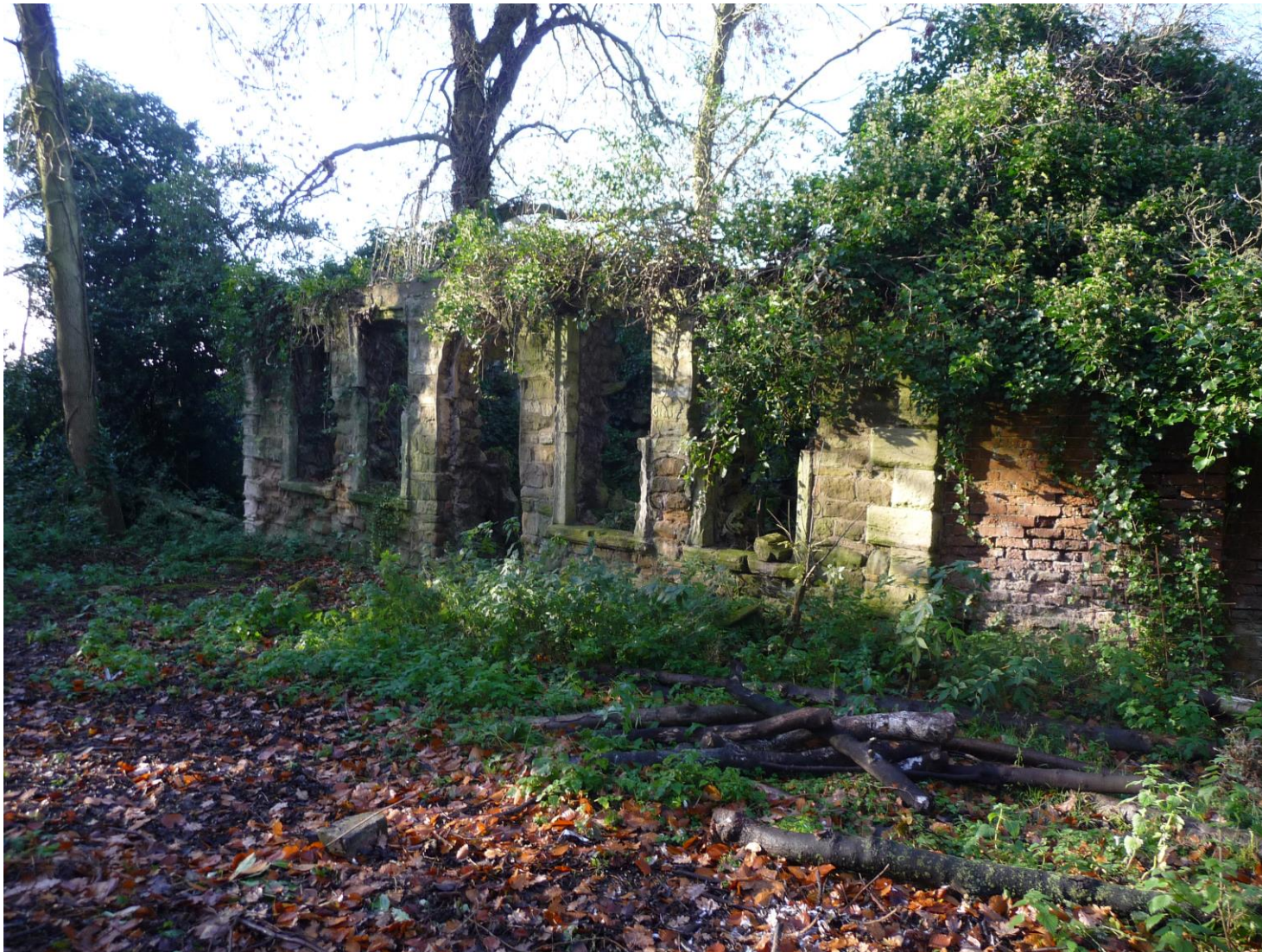
Figure 8 - Photograph of the former Orangery and possible aviary/fernery taken in 2010
