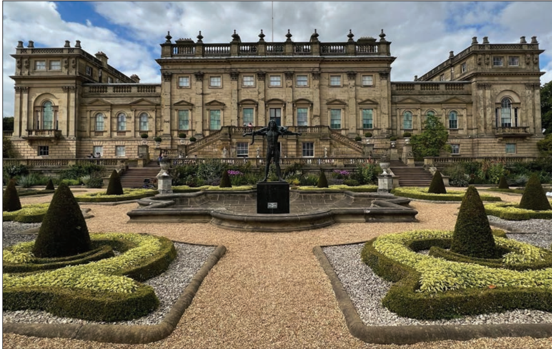
Harewood House – South Front and Parterre (Image © Gail Falkingham.)
