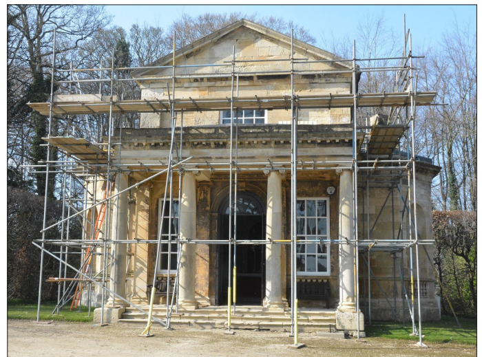
Chapel at North End of Terrace under restoration
