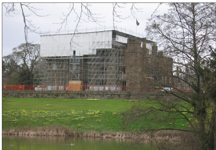
Ripley Castle roof repair
