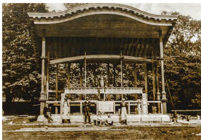
The bandstand under construction in 1914. Photo credit: Todmorden Civic Society.
