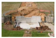
Figure 5 – New concrete liner, *photo Nick Lane Fox*
