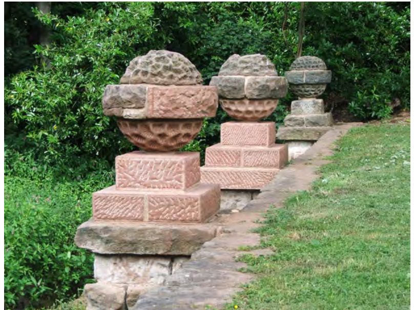
The dam (John Carr of York, 1755) with restored finials.
