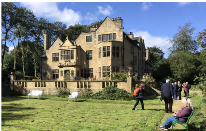
The house from the front lawn
