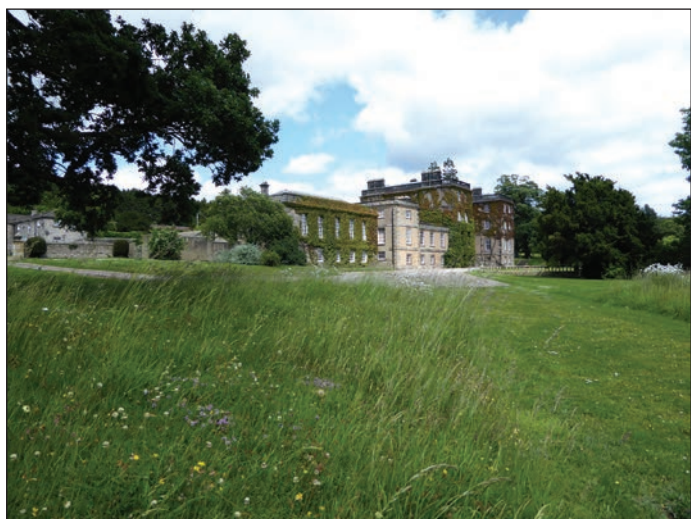
Bolton Hall from SW
