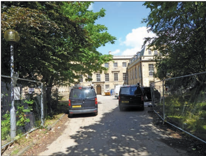
View to High Melton Hall Entrance Front from south
