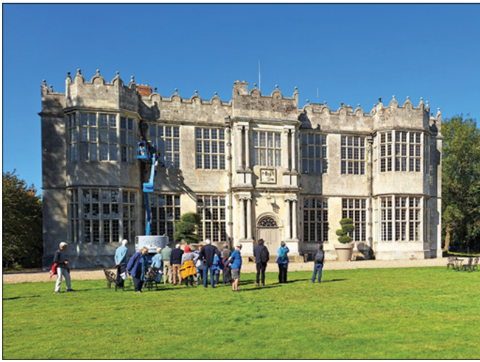
Members inspect the south front of Howsham Hall
