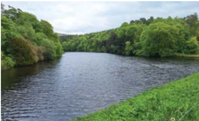
View to the north of Ingleborough dam from the 1830s dam
